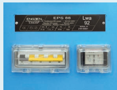
4 Circuit breakers plus ELCB protection
