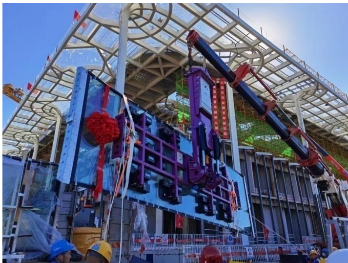
DRS 5T heavy glass installation
