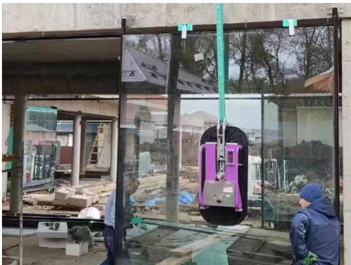
Glassboy for glass installation
