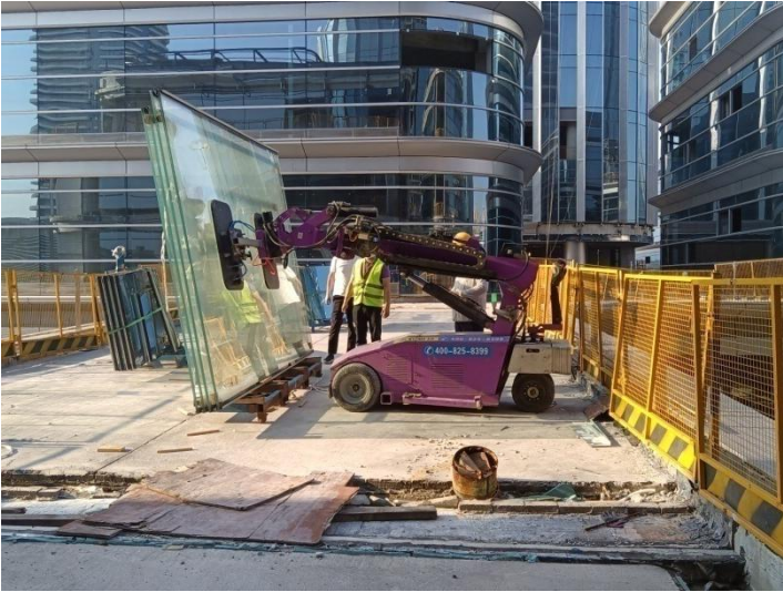
WSR 800L Pavilion installation
